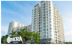
Flora An Dao (Completed) Location: Ho Chi Minh City Type: Condominiums Total Units: 500 Completion: 2016
